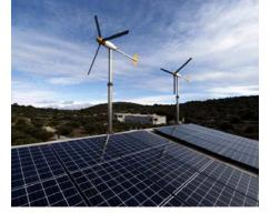
Although they must self-align with the wind, Horizontal Axis Turbines are mechanically simple and require a relatively small foundation and guy wires on the ground to mount and secure the tower.
