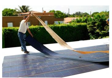
roof top. Saving you the cost of regular shingles or steel roofing, thin film solar panels are a good choice.
