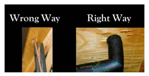
Attic wire penetrations must be secured. Insulation on right is glued and mitered. Note that insulation abuts roof decking and does not penetrate it. The hole through the deck must be caulked.
