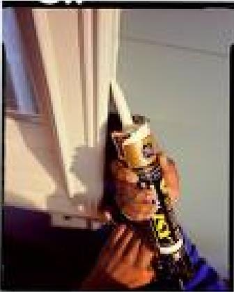
Don't forget on a sunny day to also seal the outside of the windows as well. Use an outside sealant for this job.
