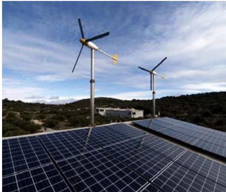
Although they must self-align with the wind, Horizontal Axis Turbines are mechanically simple and require a relatively small foundation and guy wires on the ground to mount and secure the tower.
