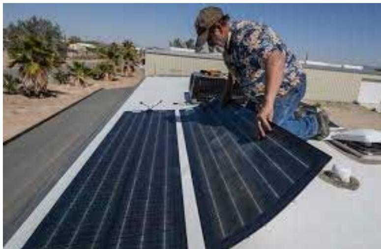
The main consideration is the type and size of wire. For example, the array wiring must be suited for outdoor use and be sized properly in order to carry the peak current.
