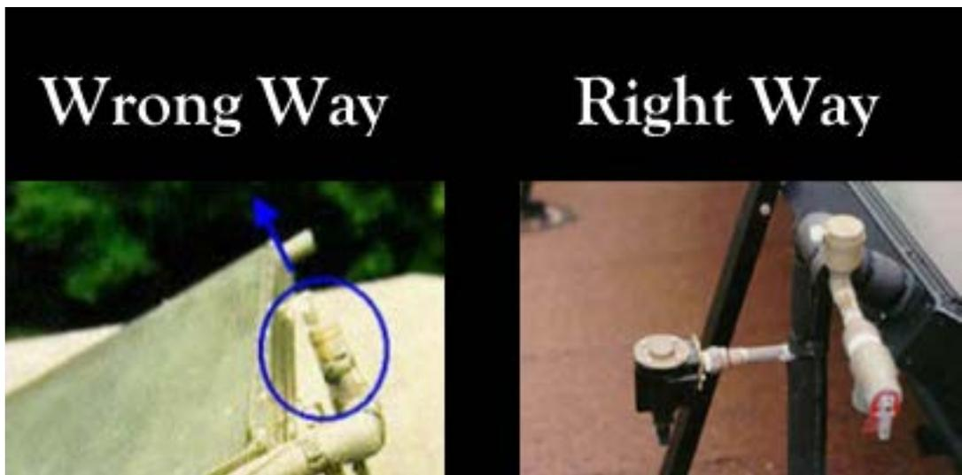
Install air vents in a true vertical position.
