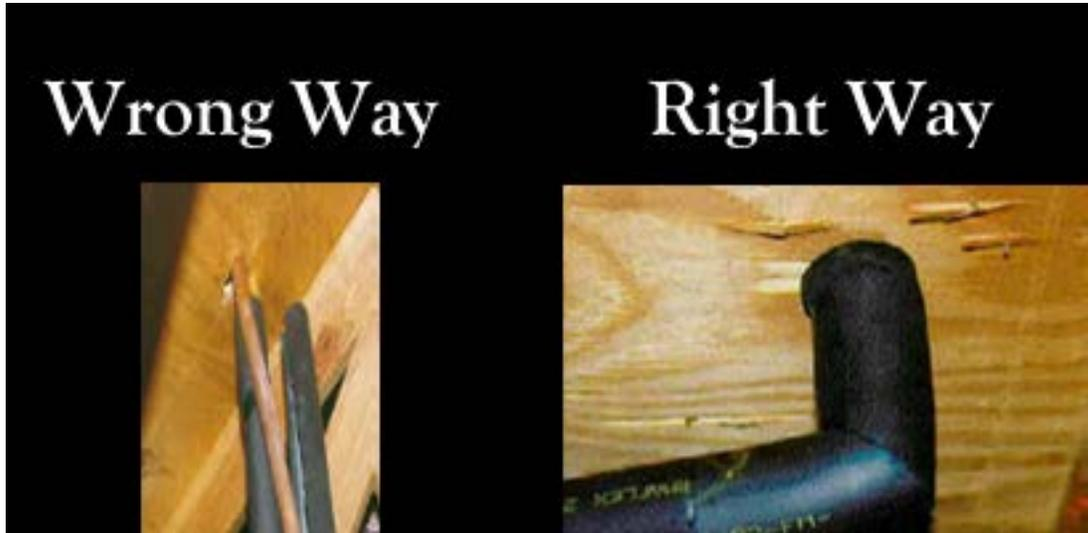
Attic wire penetrations must be secured. Insulation on right is glued and mitered. Note that insulation abuts roof decking and does not penetrate it. The hole through the deck must be caulked.
