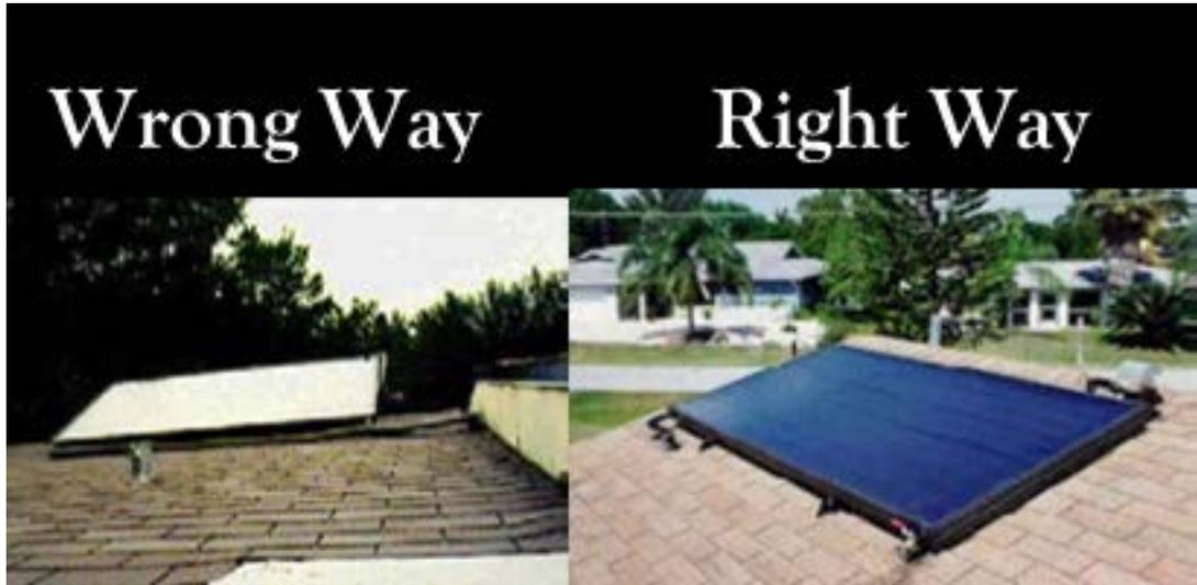
Efficient roof placement of your solar panels minimizes pipe runs and keeps pipes sloping downward. Keep pipe runs should be less than 20 feet if possible.
