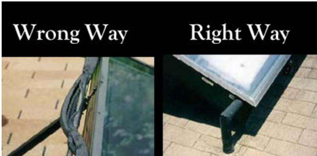
All wires exposed to the weather should be jacketed with PVC pipe, or aluminum, or painted.
