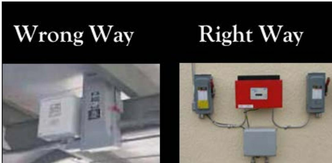
Service providers must be able to disconnect each piece of serviceable equipment in the PV system, such as arrays and inverters. In simple systems there will be a DC disconnect between the modules and the inverters and an AC disconnect between the inverters and the panel. Components need to be placed in readily accessible locations.
