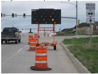
The alpha numeric signs you see that flash words and numbers are usually solar. In the old days these bulbs used in the sign to make the flashing arrows used to be powered by small combustion engines. Not anymore.
